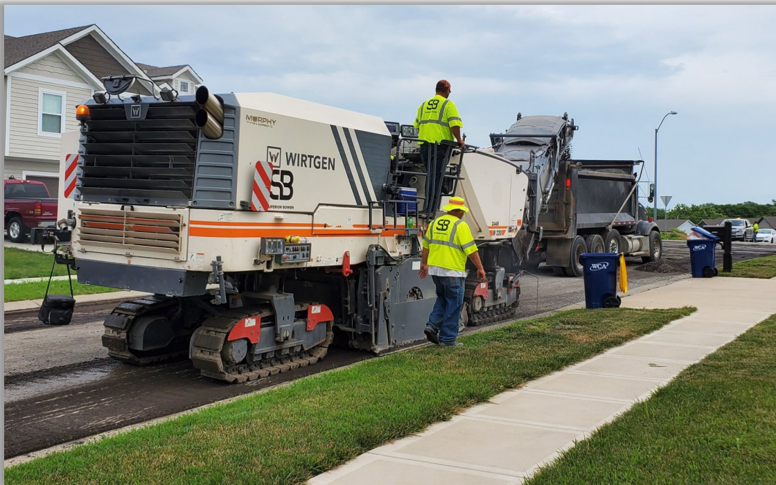
Contracted construction workers finish mill and overlay on a neighborhood street in the Rock Creek Subdivision in 2021
